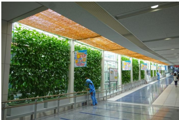
Green Curtain (Terminal 1 passage)
