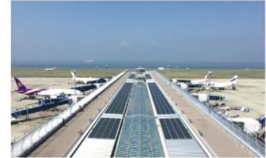
Solar power generators (Terminal 1 Bldg.)
